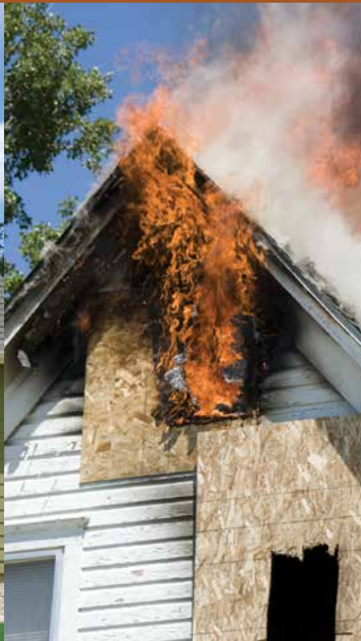
Residential Attic and Exterior Fires
